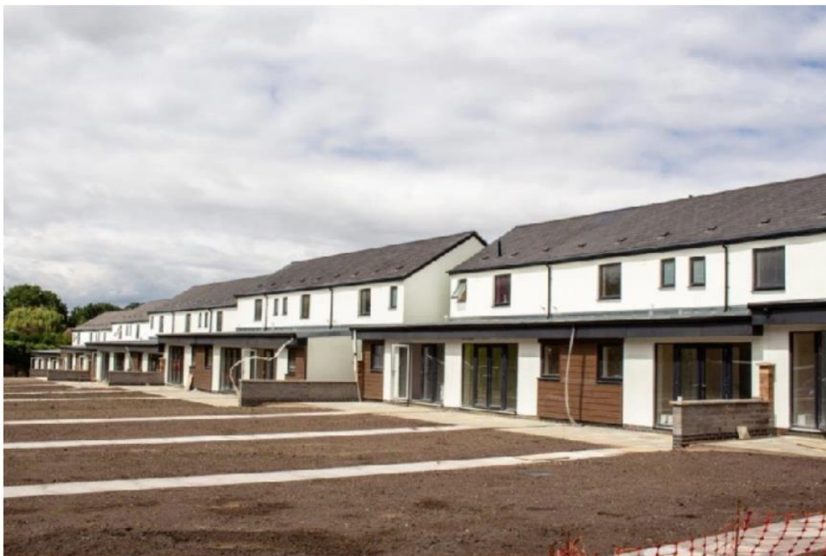
Some of the refurbished homes on Newfield Road. EMN-190618-174220001
