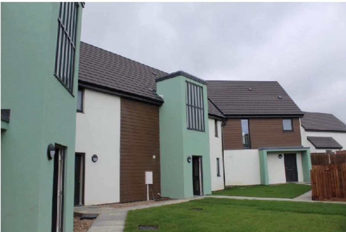
Newly built homes on Newfield Road. EMN-190618-174256001
